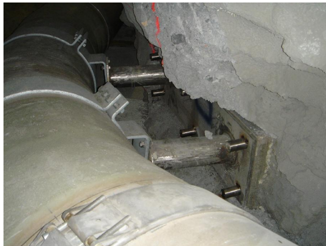
Protection against centrifugal and axial forces
