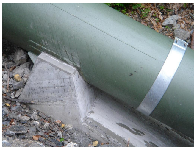
Protection against centrifugal and axial forces
