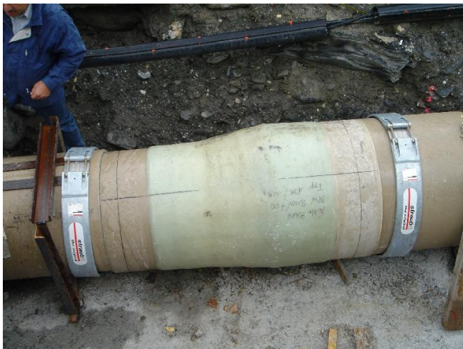
Clutching of pre fabricated laminated transition pieces
