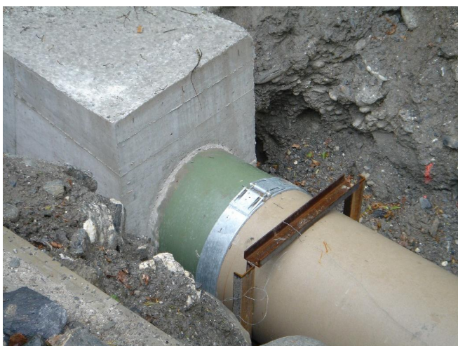
Clutching of pre fabricated laminated transition pieces
