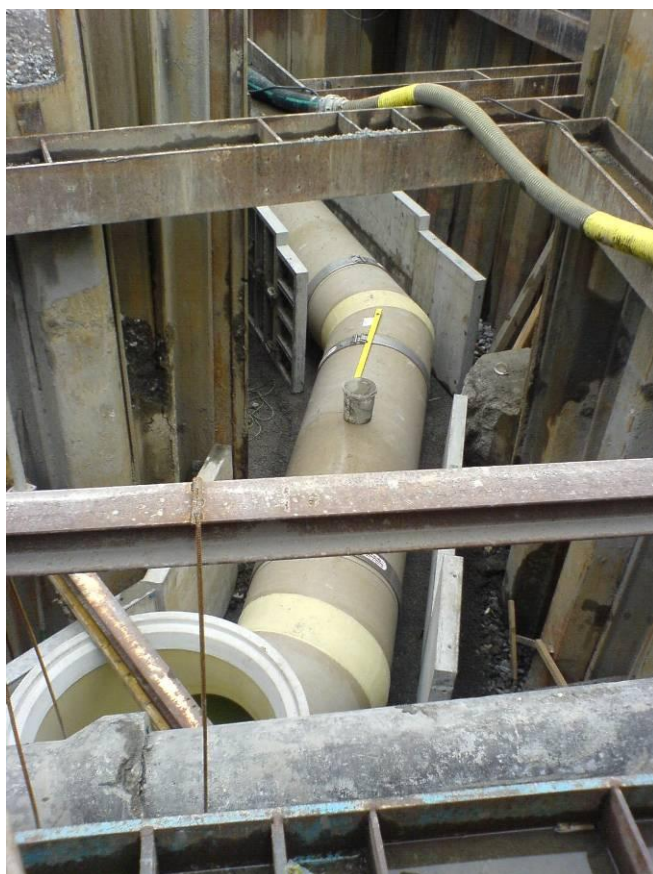
Picture : left Finished assembled HOBAS tubes and HOBAS "Man Hole" piece
