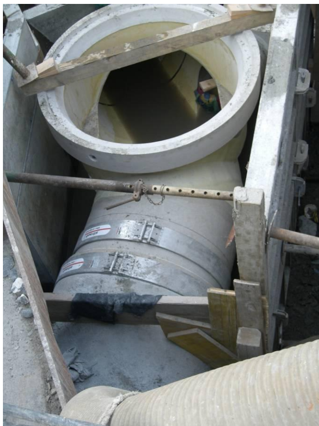
Picture: upon Intermediate piece to connect HOBAS tube DN 1000 with existing asbestos tube
