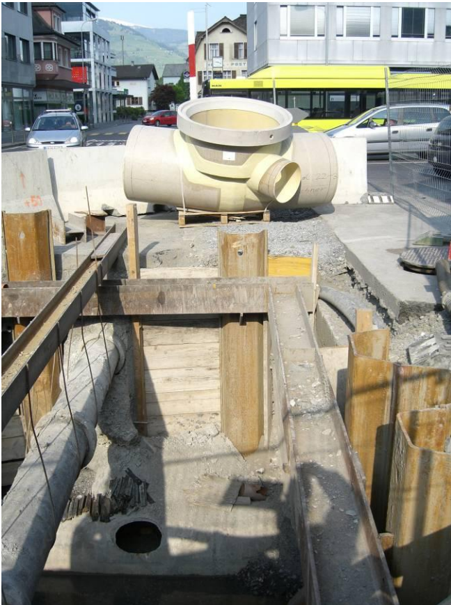
Picture: upon Intermediate connection piece between of old style asbestos tube and new HOBAS tube
