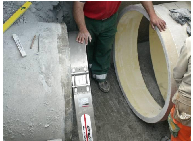
Picture: upon Intermediate connection piece between of old style asbestos tube and new HOBAS tube
