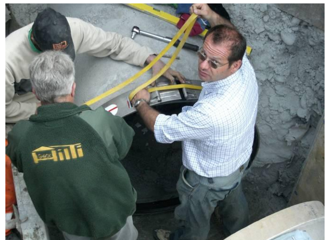
Picture: upon and left Training on place by a STRAUB Specialist connecting Asbestos with HOBAS tube by a STRAUB FLEX 2LS coupling
