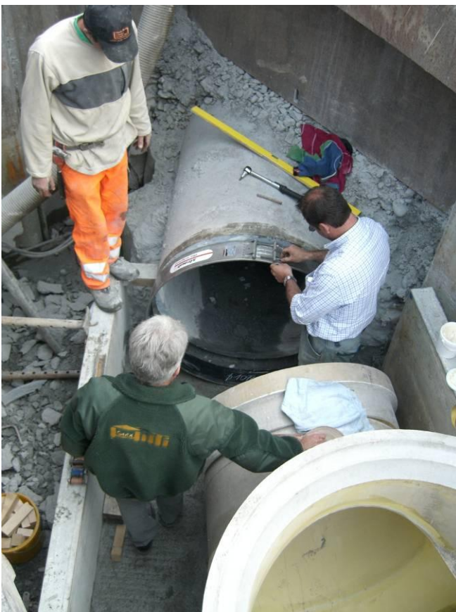
Picture: upon and left Training on place by a STRAUB Specialist connecting Asbestos with HOBAS tube by a STRAUB FLEX 2LS coupling
