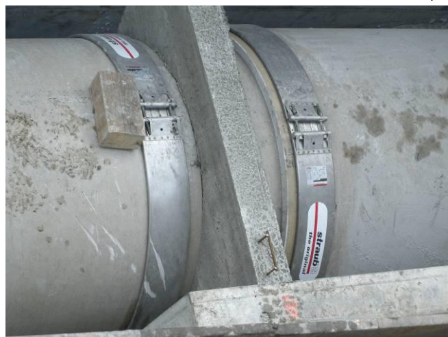
Picture: upon Intermediate piece to connect HOBAS tube DN 1000 with existing asbestos tube
