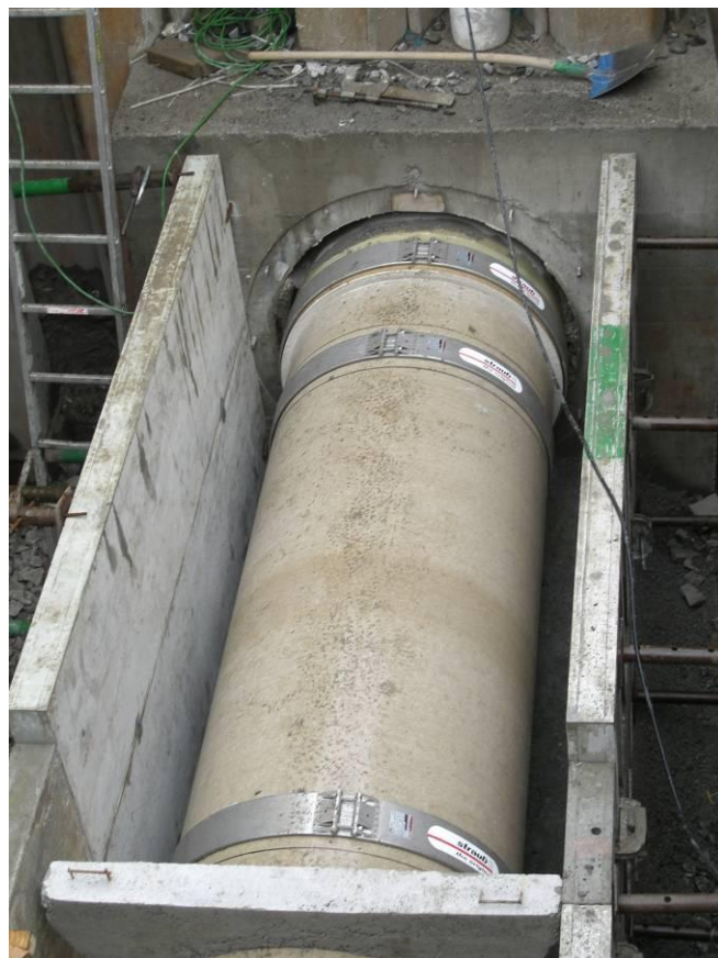
Picture: left Mounted HOBAS “Man Hole” piece with intermediate piece and STRAUB-FLEX-2LS coupling
